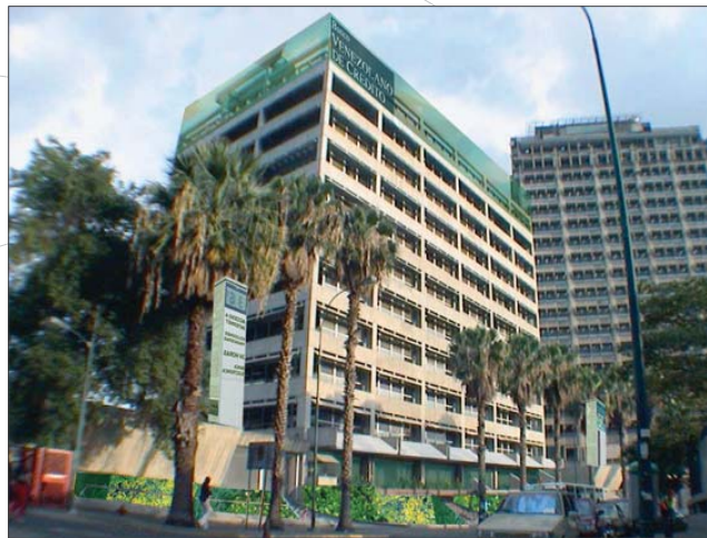
main facade view
